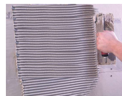
TILE ON DRY WALL BOARDS
