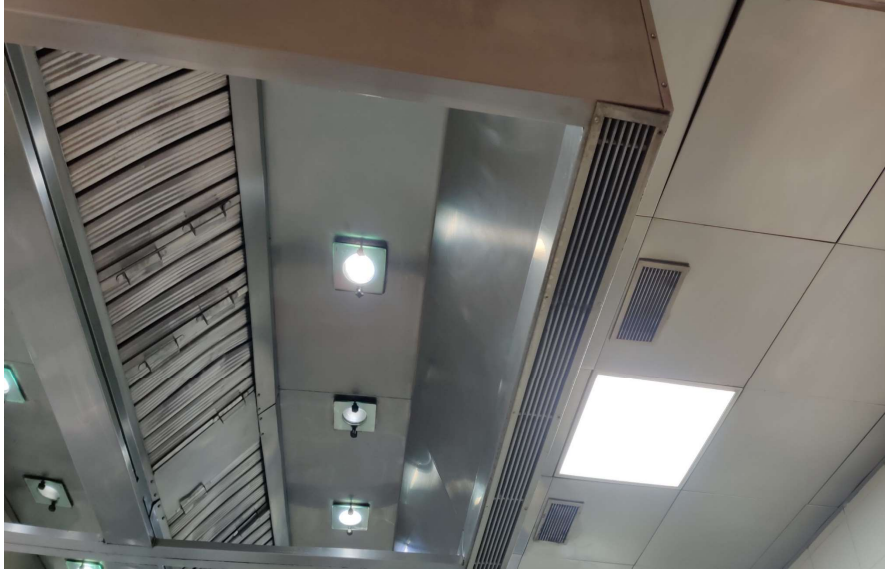
Kitchen – Part Section Showing Exhaust, Compensatory Air and TFA Outlets
