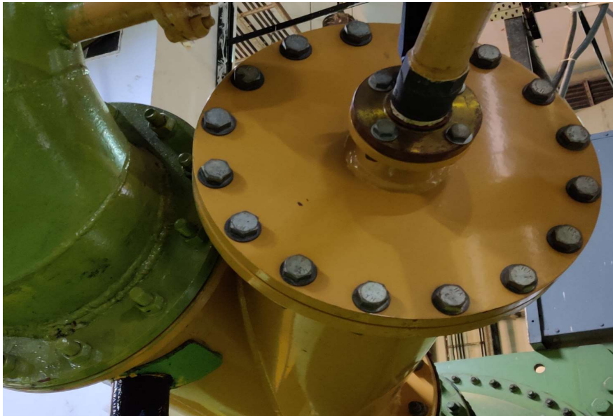
ATCS Fitted to Chiller
