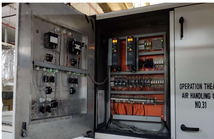
Factory Fitted VFD on Air Handling Unit
