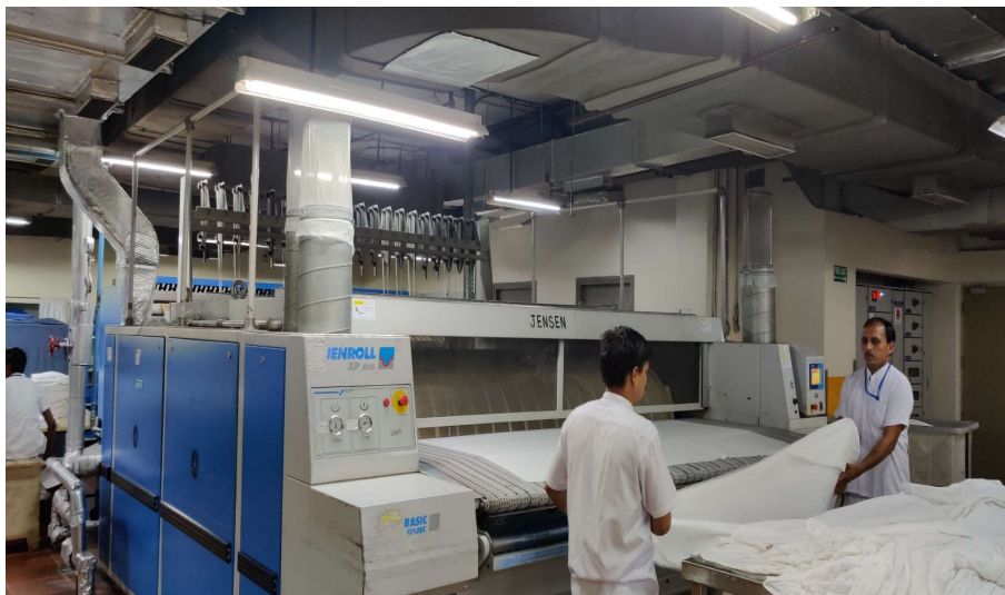
Air distribution Above Flat Work Ironer
