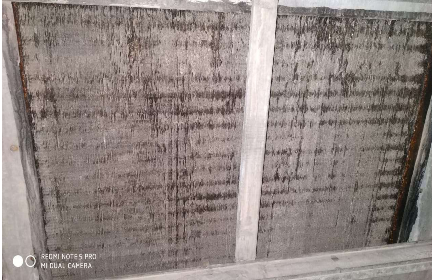
Air Handling Unit without U.V Tubes
