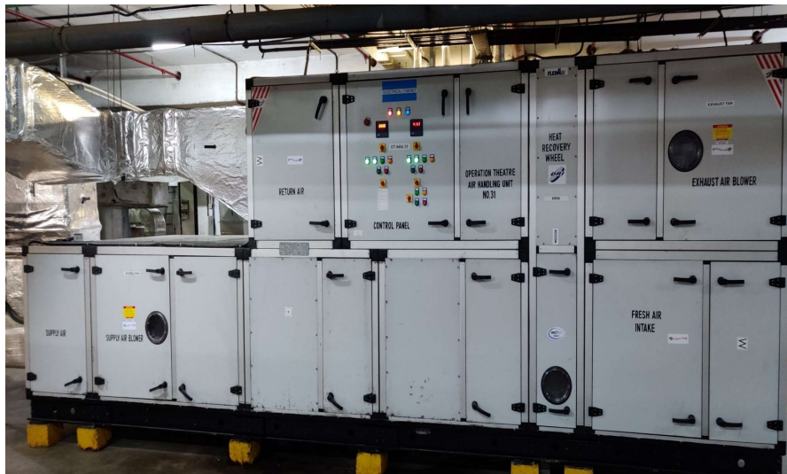
Factory Fitted VFD on Air Handling Unit
