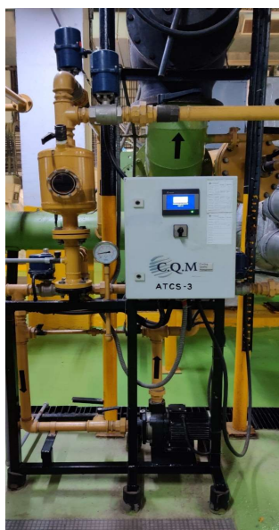
ATCS Fitted to Chiller
