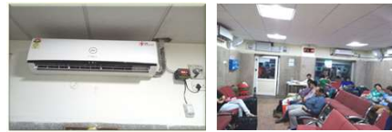
Inverter type AC units in Waiting halls
