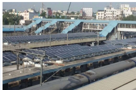
500 kWp On Grid plant on RCC rooftop of PFs at SC stn.
