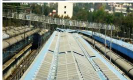
227.5 kWp On Grid plant on Galvalume sheets of PFs at HYB stn.
