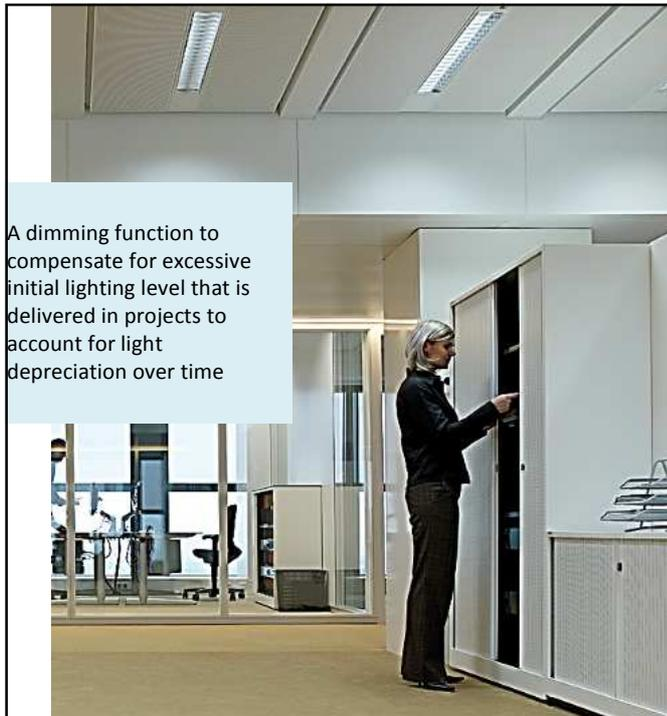
A dimming function to compensate for excessive initial lighting level that is delivered in projects to account for light depreciation over time
